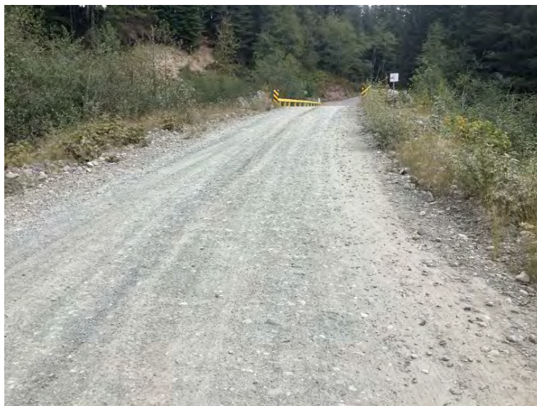
Approach from Right Bank when facing downstream
