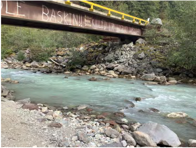
Left Bank Abutment when facing downstream
