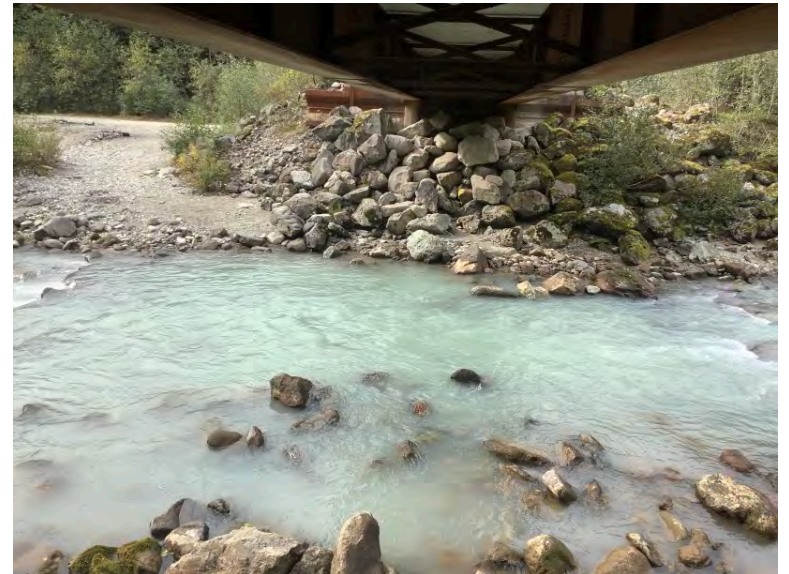
Right Bank Abutment when facing downstream
