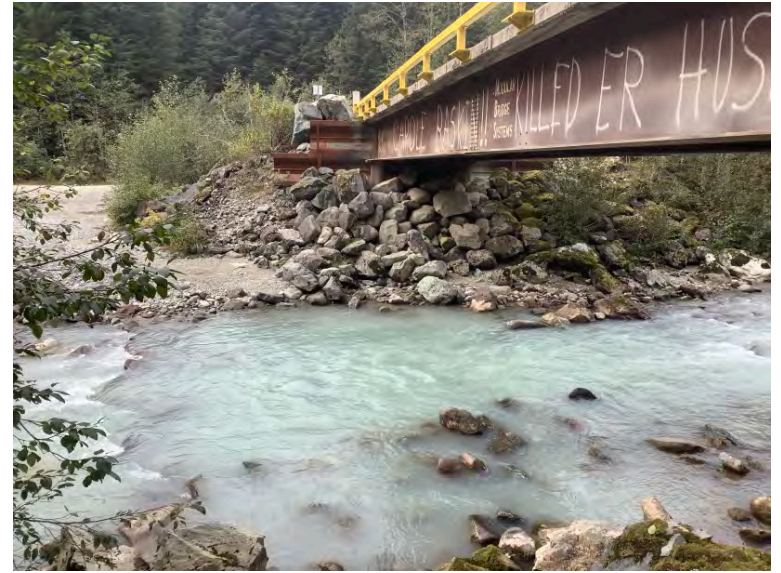
Right Bank Abutment when facing downstream
